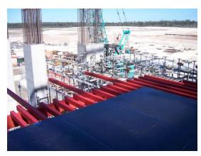
This product is designed specifically for use as concrete formwork. Formply, due to its short life as a structural member as concrete formwork, may be manufactured to either the structural plywood Standard AS/NZS2269 with Type A bond and B grade or better faces on two sides, or bonded to the exterior plywood Standard AS/NZS2271 with Type B bond or the interior plywood Standard AS/NZS2270 with a Type C bond and B grade or better faces both sides.
