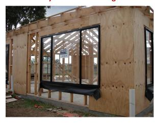
Structural plywood manufactured to AS/NZS2269, normally a minimum of DD grade, provides a simple but reliable means of bracing building framing against wind and earthquake damage. Structural plywood claddings and linings with A grade faces can perform the dual functions of being aesthetically pleasing and structural bracing.
