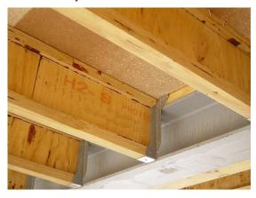
Glued I-beams utilising structural LVL's high tensile and compressive strength in flanges, and plywoods high panel spear capacity in the webs, provide an economical, structurally efficient beam. These composite beams are generally used as floor joints or purlins with each manufacturer providing specific design data.
